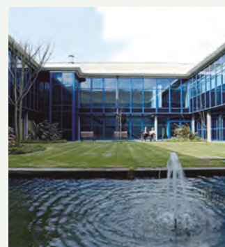
NHS Canford house clinic, Bournemouth, UK. VRF
